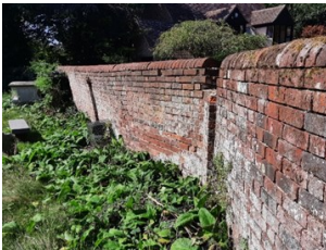
The wall before demolition
